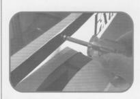
Use two screws to secure the hatch firmly.
